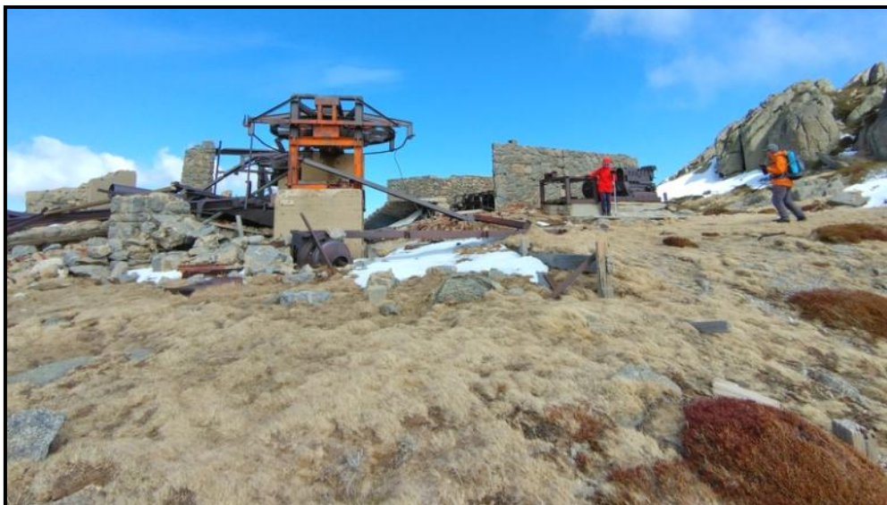
At the Stilwell restaurant ruin, Monday 23 September 2024. Photo: Garry Boxsell
