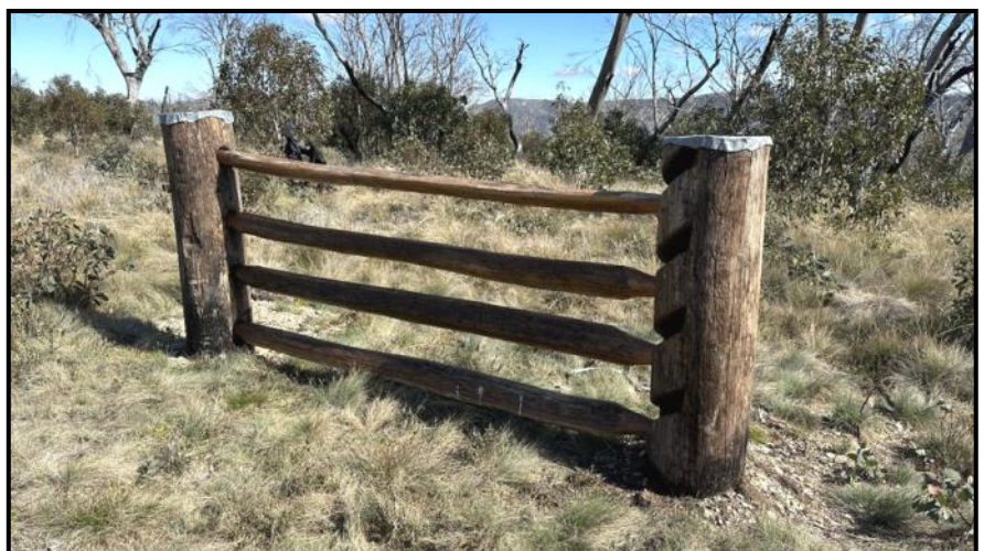
The newly rebuilt sliprail at Four Mile Saddle. Photo: Alan Levy
